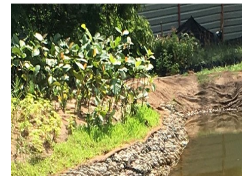
Geotextile with turfing
