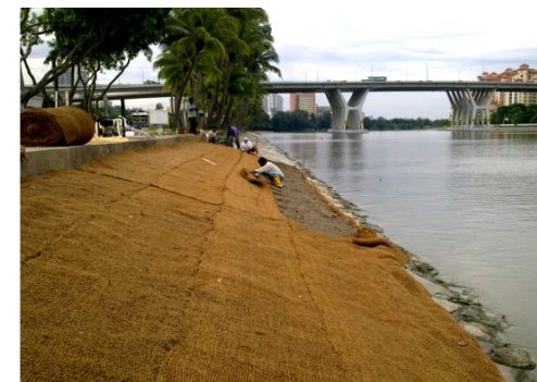
Laying of coir webbing on the soil before plants establishment
