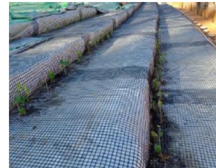
Slope Reinforcement
