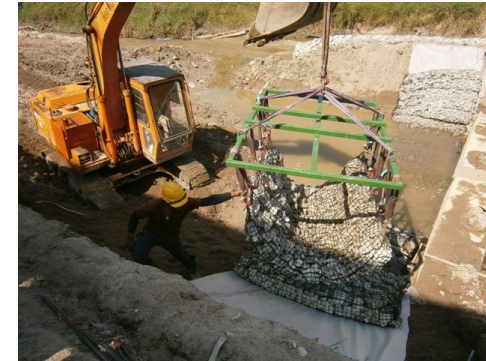
Lifting of rock chamber mattress
