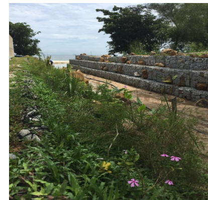
Bio- engineered Slope
