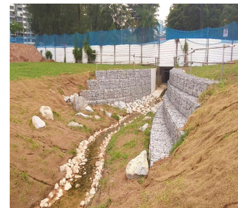
Bioengineered slope
