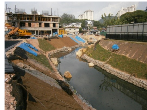
Bio-engineered slope
